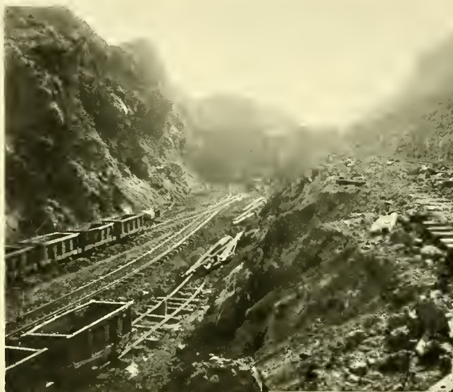
MINING IRON ORE IN OPEN CUT AT ORISKANY, • CRAIG COUNTY, VA.
